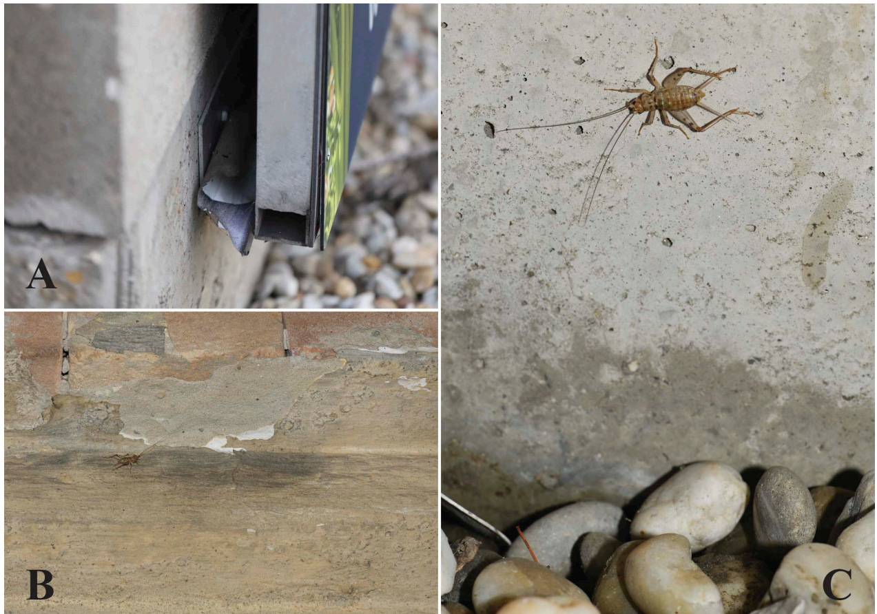
Figure 4. Microhabitat of the alien G. dalmatina outside its native range. A: detailed view on the 4 cm narrow space between the billboard and building. B: Detail on the old building wall with the typical insect posture. C: Lining of buildings with small gravel used as a refuge especially during escape behaviour. Animals were not arranged. Photo: J. Svetlík.
