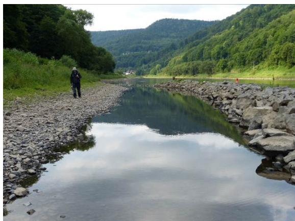
Figure 1. Elbe River at site 3, on 19 th June 2014. Man-made river groyne near Děčín. Photograph by M. Straka.
