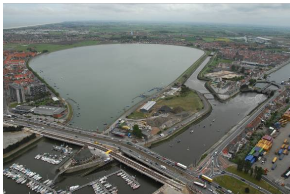
Figure 5. Aerial view of the Sluice Dock at Oostende. Photo courtesy of MUMM.
