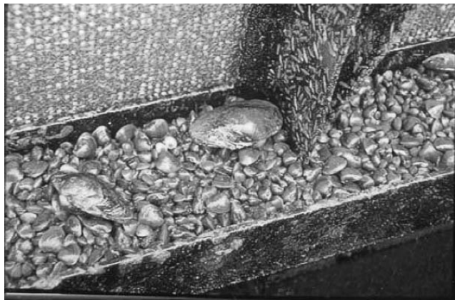
Figure 7: Asiatic clam and native unionid larvae pass through intake screen and grow to maturity on "clean" side of screen.
