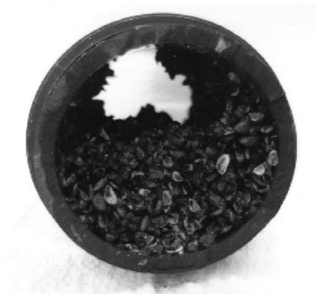
Figure 6: Zebra mussels clog 6-in. biomonitoring trailer discharge pipe after only three months.
